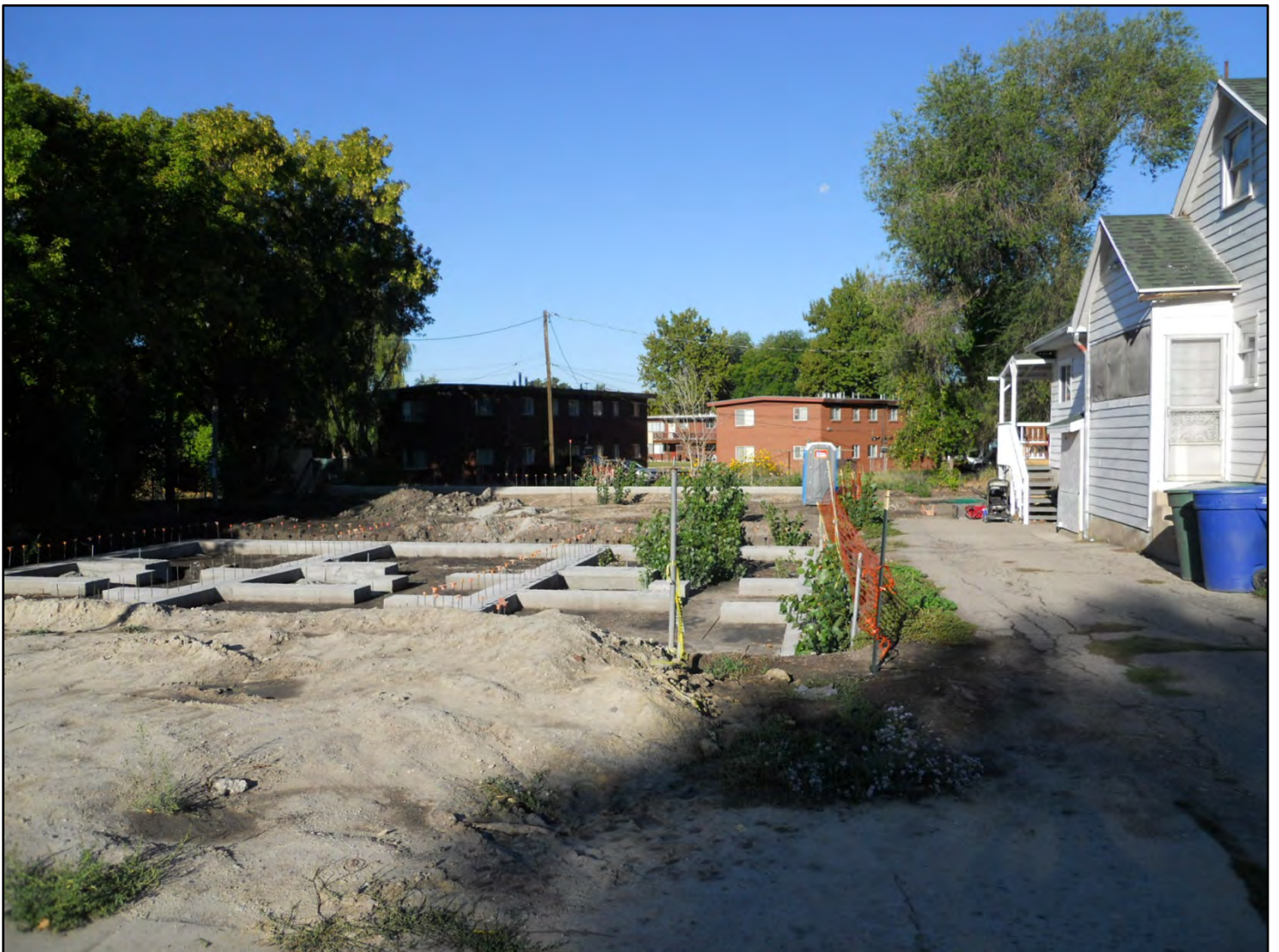
Footings for Attached Single-Family Dwelling South of Adjacent Driveway
